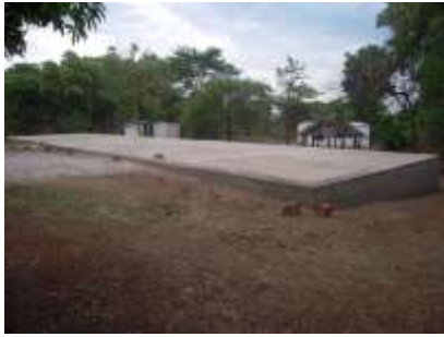
The foundation slab for the new two block classroom
